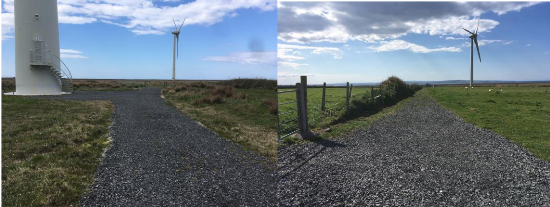
Plate 2-9: Photos of Access Tracks at Lackan
