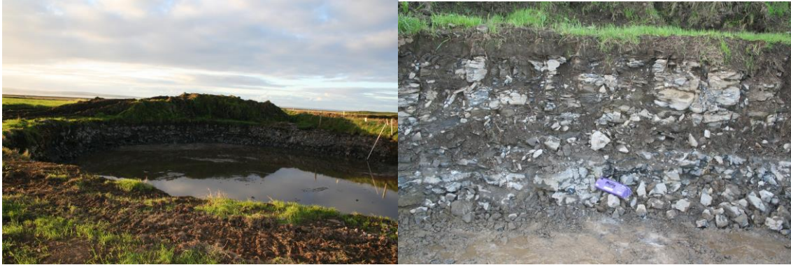
Plate 2-6: Photos of Turbine T3 Foundation Earthworks
