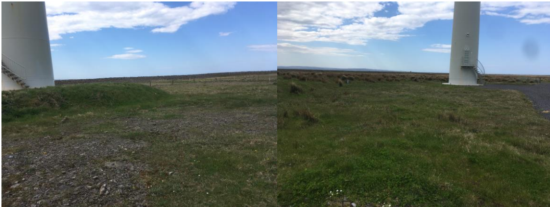
Plate 2-10: Photo of T2 and T1 Hardstands
