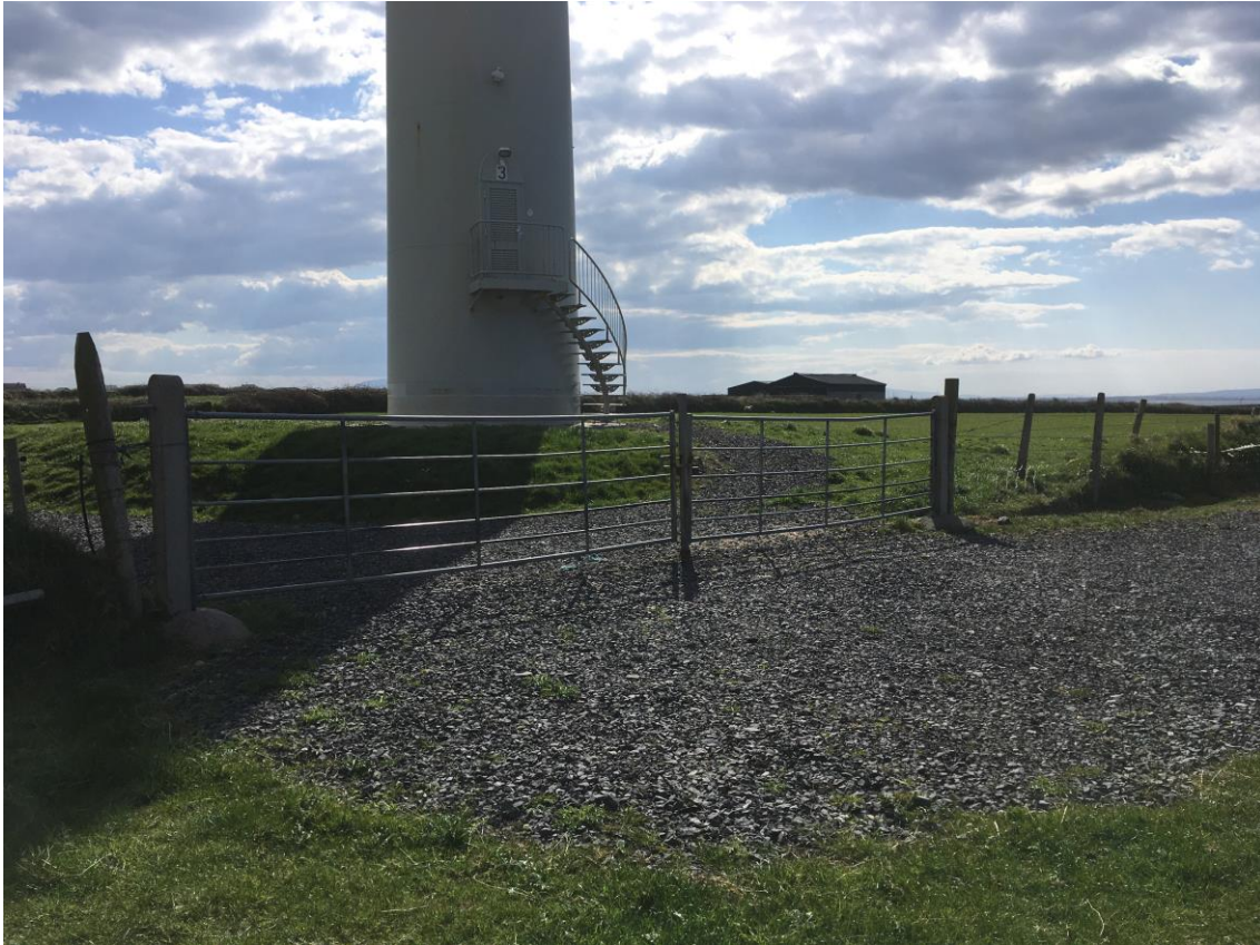
Plate 8-3: View of General Topography – Turbine T3
