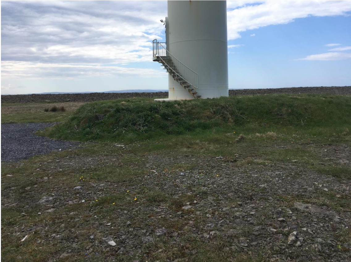
Plate 8-1: View of General Topography – Turbine T1
