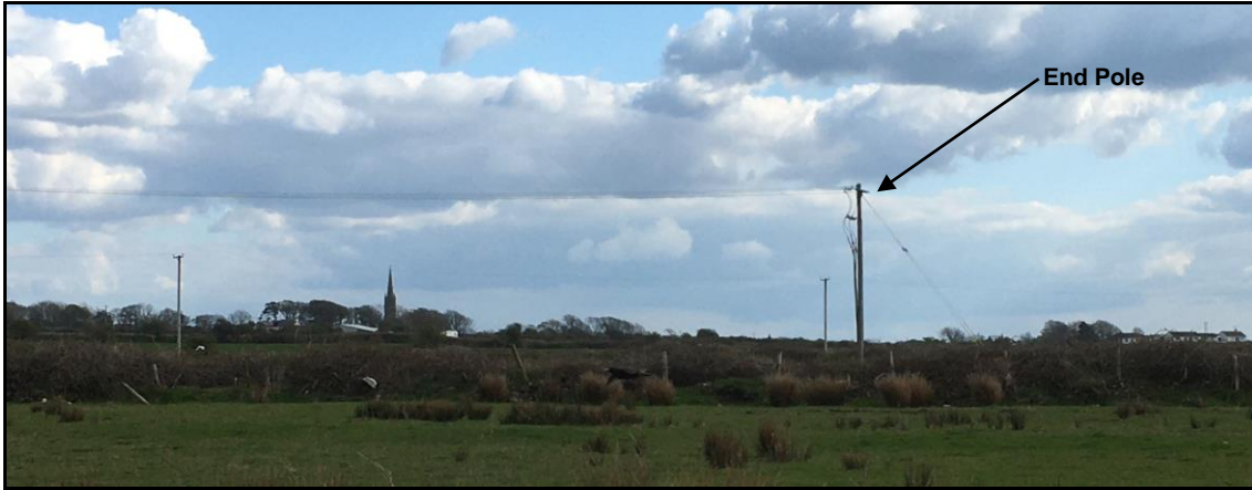
Plate 2-12: Grid Connection End Pole Looking South from L6502
