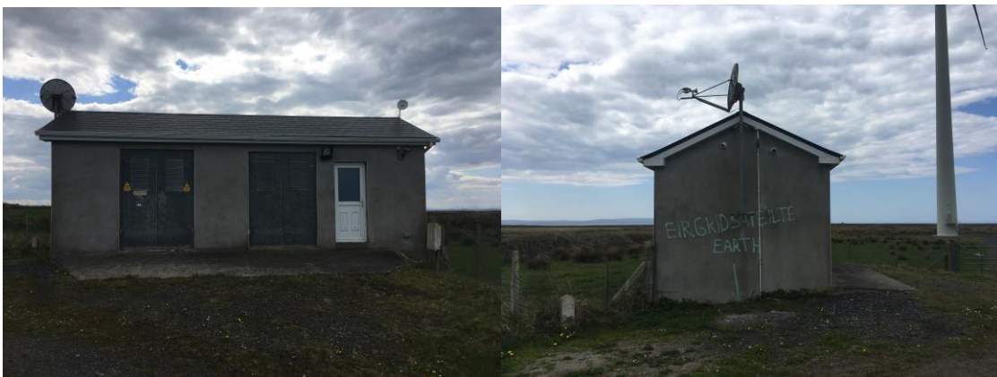
Plate 2-8: Photos of Lackan Control Building
