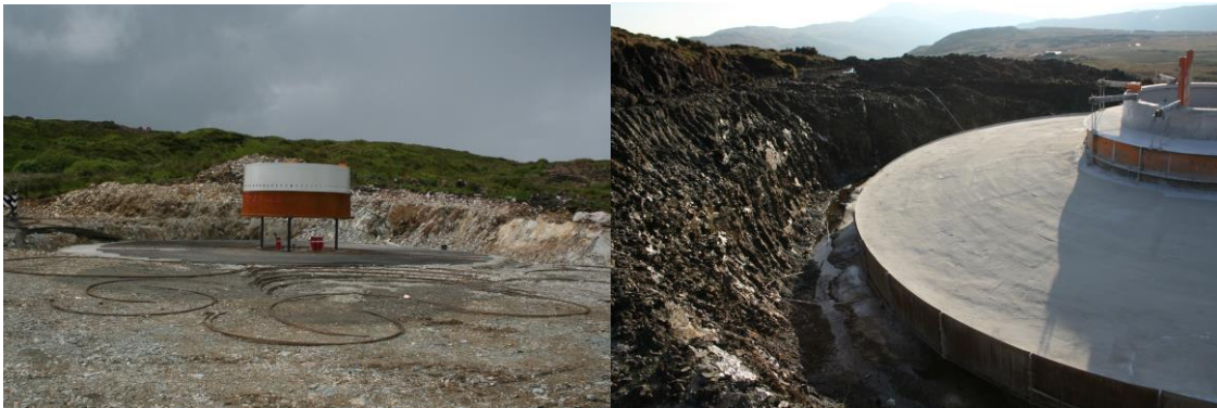
Plate 2-7: E70 Foundation Construction Photos
