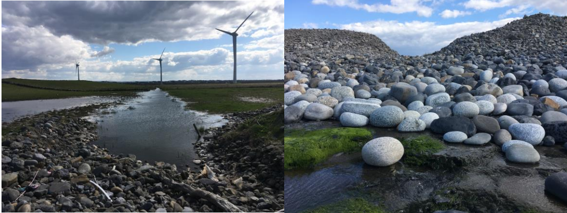
Plate 7-5: Drain & Culvert Through Dyke – Northern Discharge
