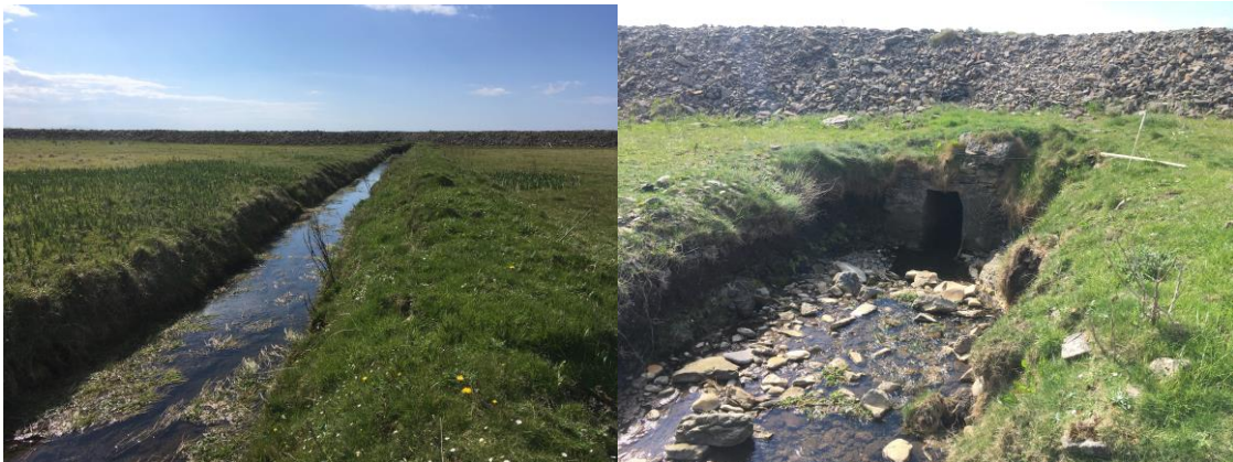
Plate 7-3: Drain & Culvert Through Dyke – Southern Discharge
