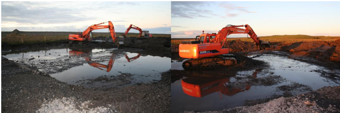
Plate 2-4: Photos of Turbine T1 Foundation Earthworks
