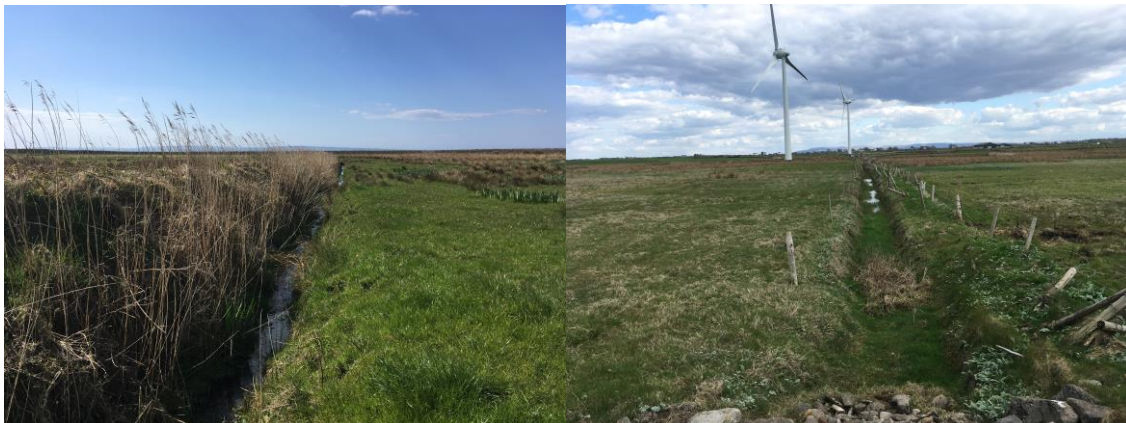
Plate 7-4: Drain & Culvert Through Dyke – Central Discharge
