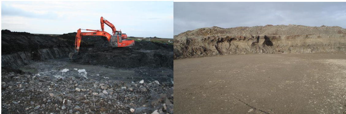
Plate 2-5: Photos of Turbine T2 Foundation Earthworks
